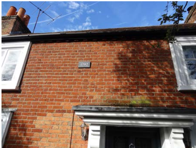
The brickwork around the front door
